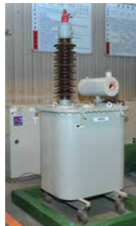
AC耐壓試驗 Separate-source AC withstand voltage test
