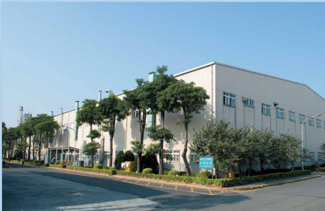
新港廠 Shin Kang switchgear plant
