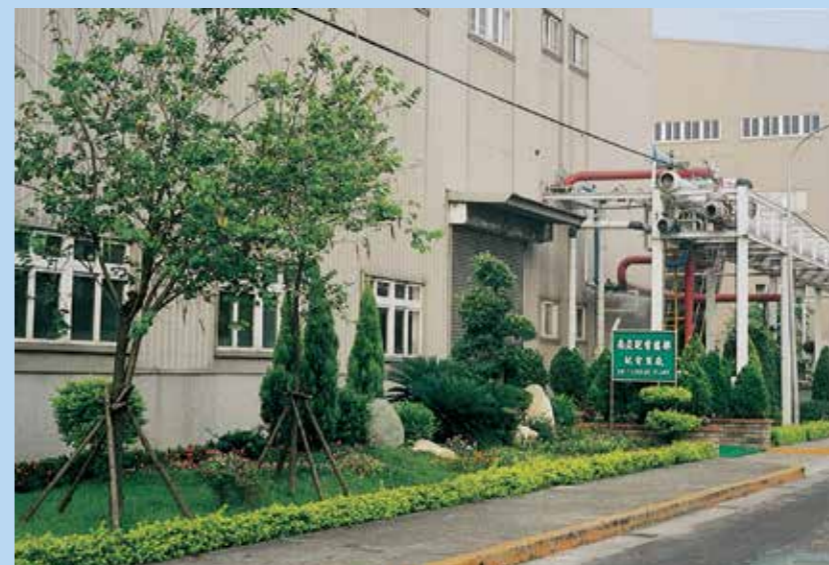
新港廠 Shin Kang switchgear plant
